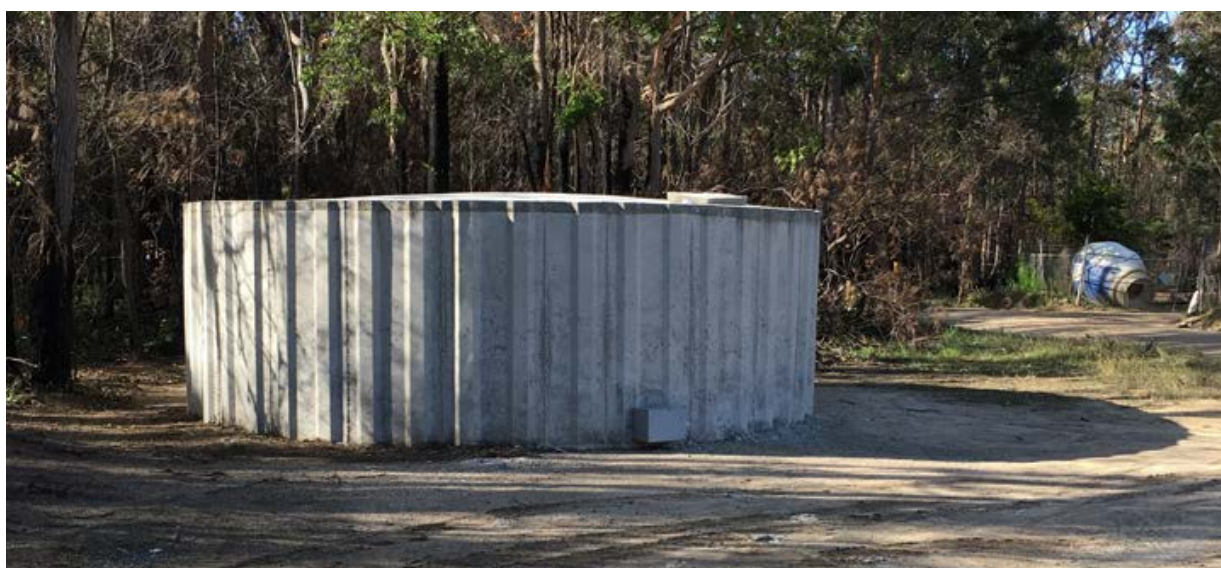
46,000L concrete static water tank in Mallacoota
