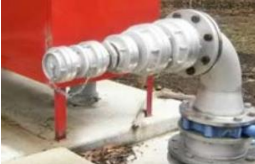
125mm, 100mm, 90mm, 75mm, 65mm Storz tree adapters.
