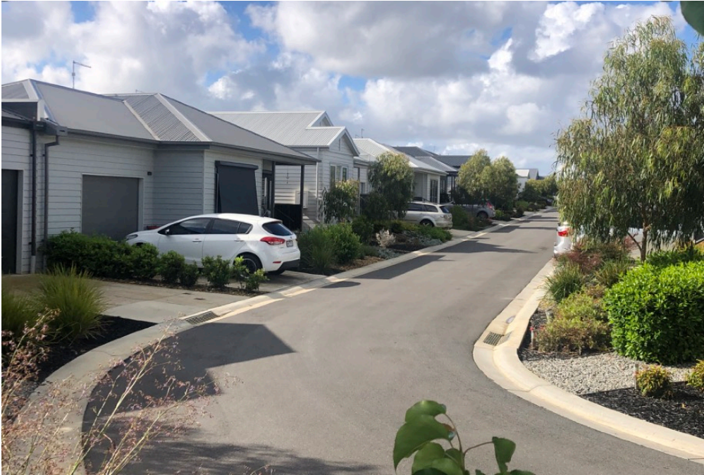
Figure 4. Typical Residential Village streetscape
