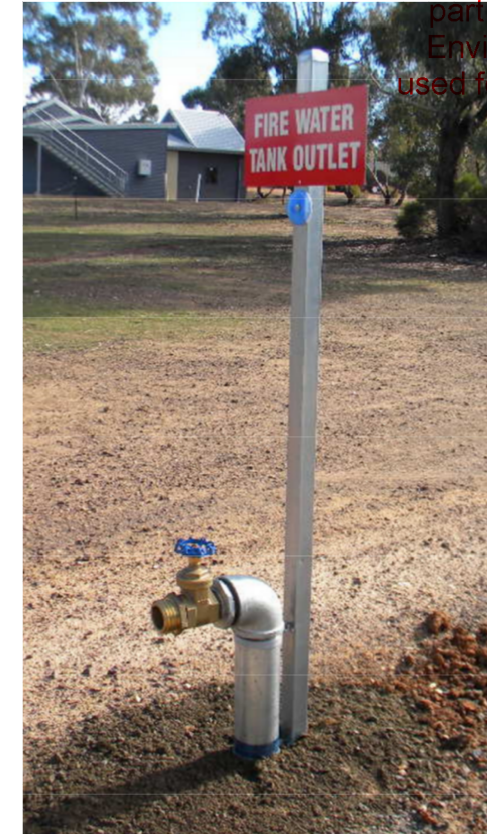
EXAMPLE OF CFA ONLY REMOTE OUTLET
