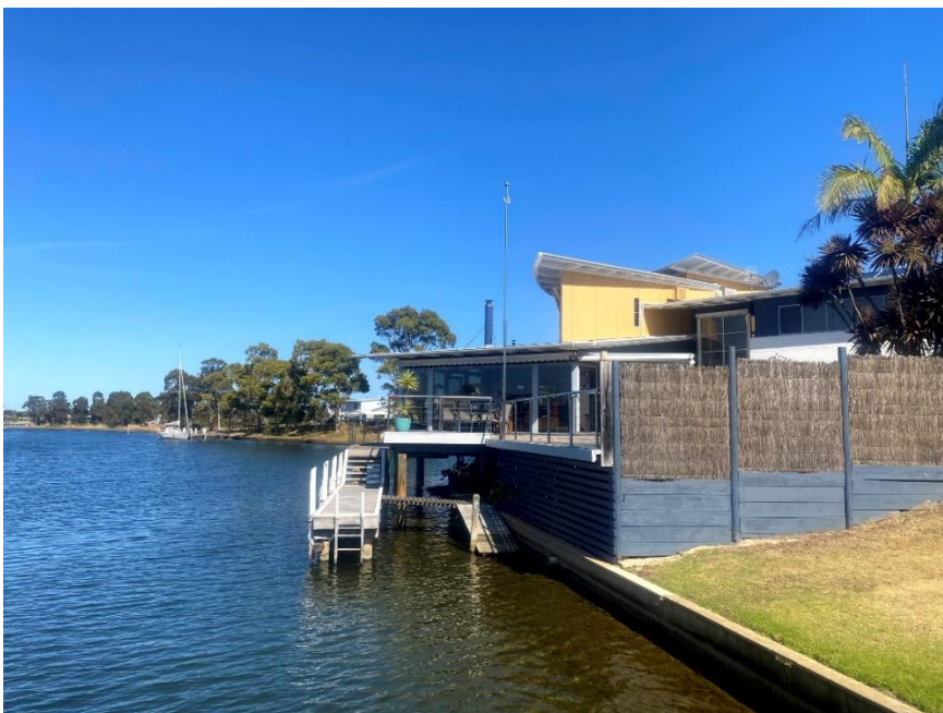
Image of 35 Canal Road, Paynesville from the subject land's jetty
