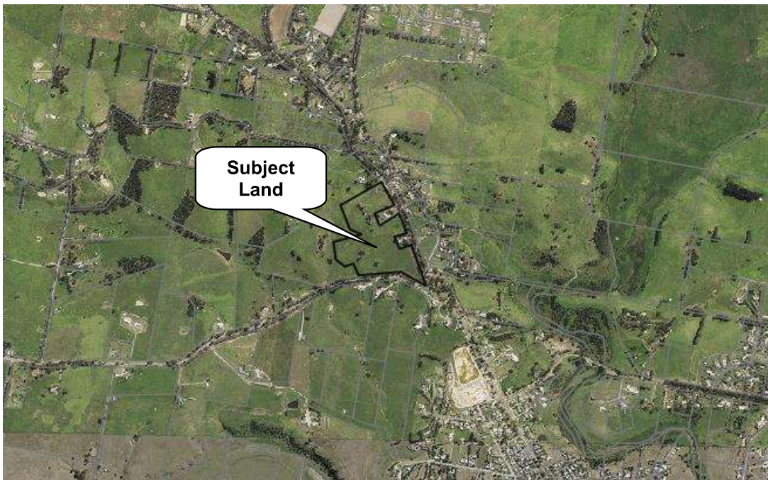
Aerial view of subejct land and surrounding precinct – Source: LASSI SPEAR (DELWP)
