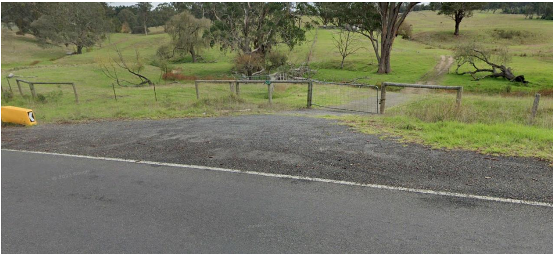
Image of the existing access to the subject land
