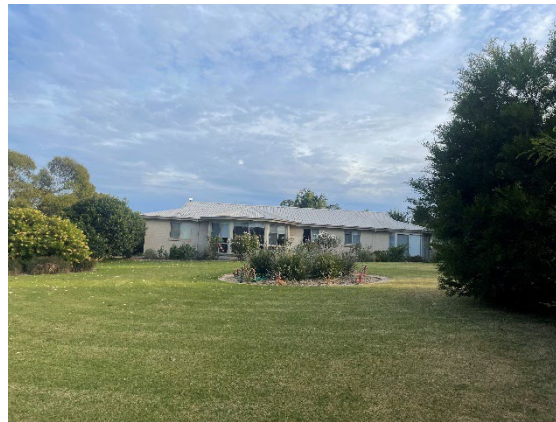
Photograph 5 – Proposed Lot 1 facing north.
