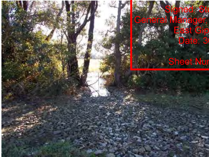
View of runoff discharging into Ward Street
