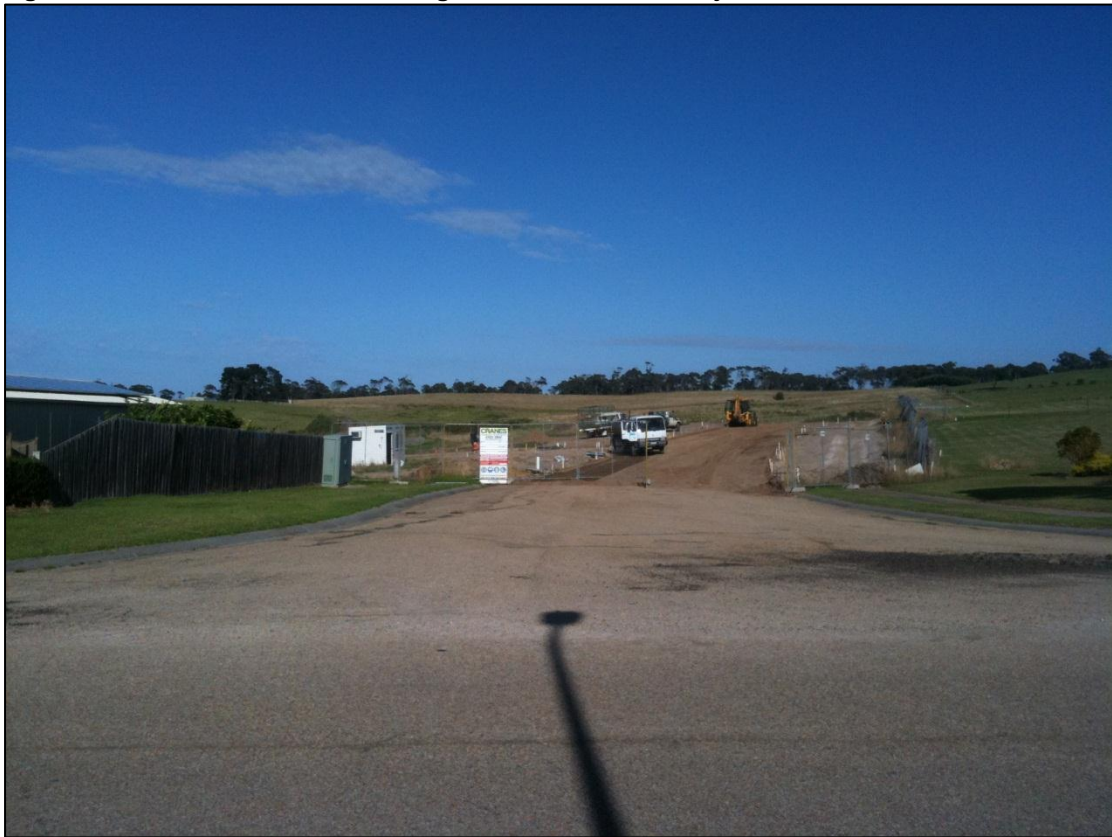
Figure 3: Lawson Drive Looking West Towards the Subject Site
