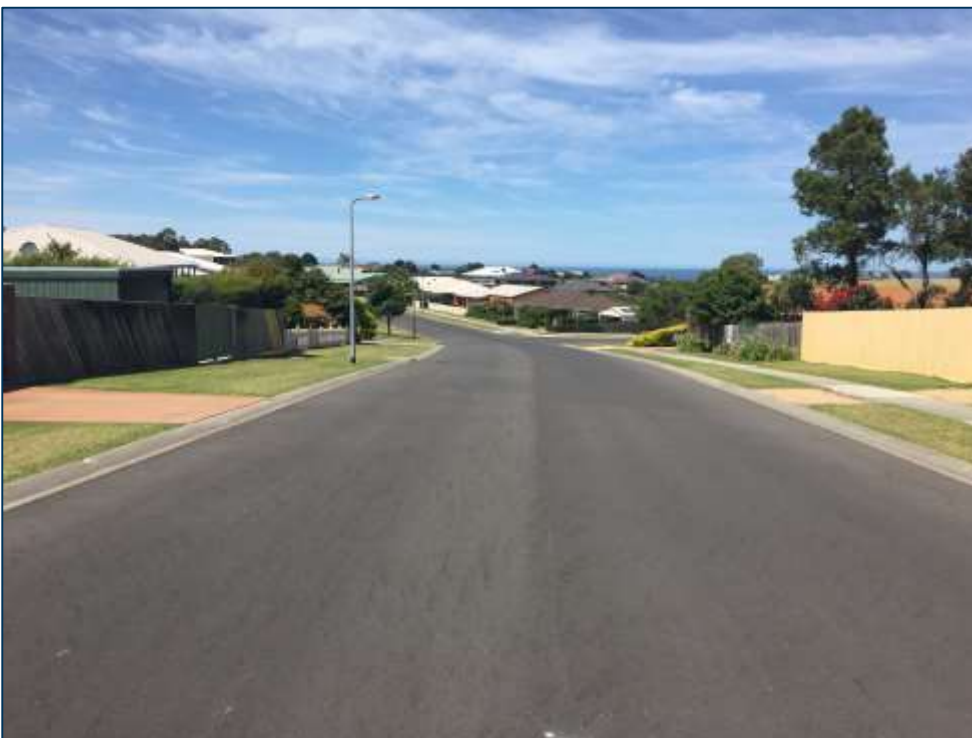
Figure 3-3 Sterling Drive looking south from Thorpes Lane towards Lawson Street
