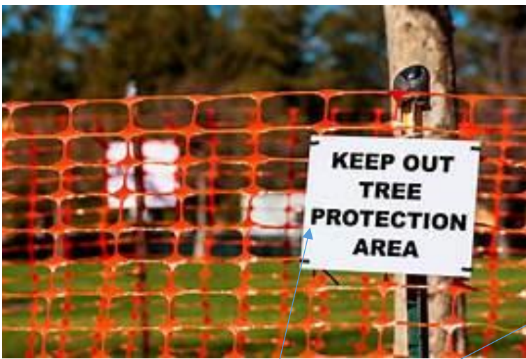
Tree Protection Fencing. Trees on development site protection
