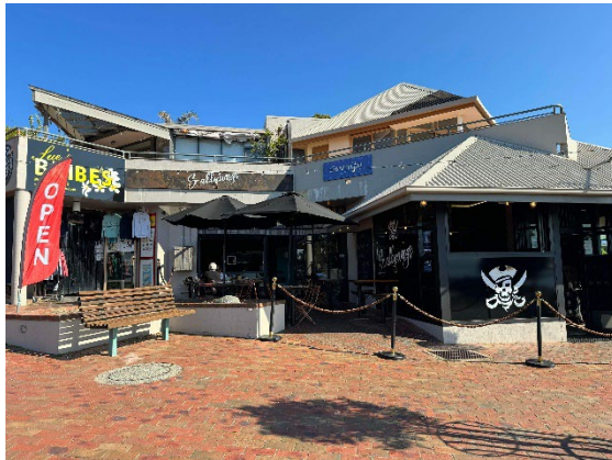
Photograph 3 – Existing commercial development on the adjoining land at 14 Allan Drive, Mallacoota facing southwest.
