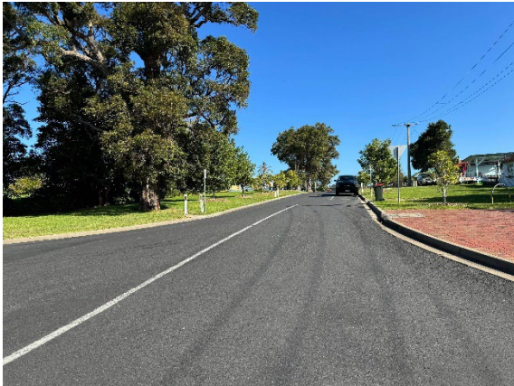
Photograph 9 – Dorron Avenue facing southwest.
