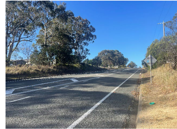
Photograph 12 – Princes Highway facing north.
