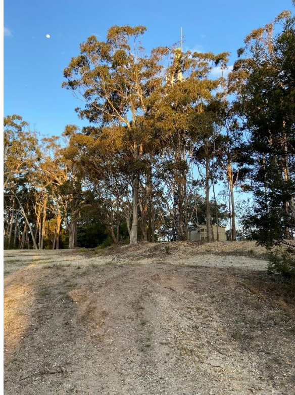
Communications tower on adjoining reserve
