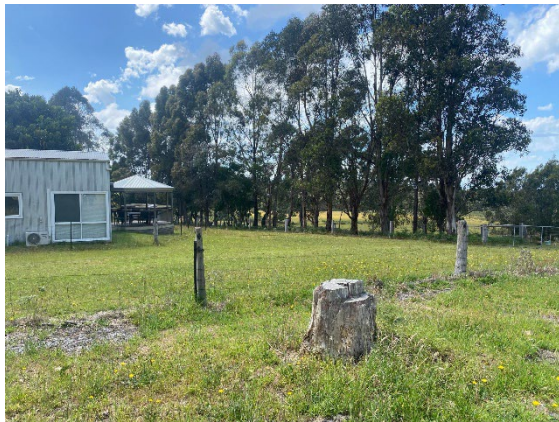
Photograph 9 – Extension to existing dwelling facing southeast.
