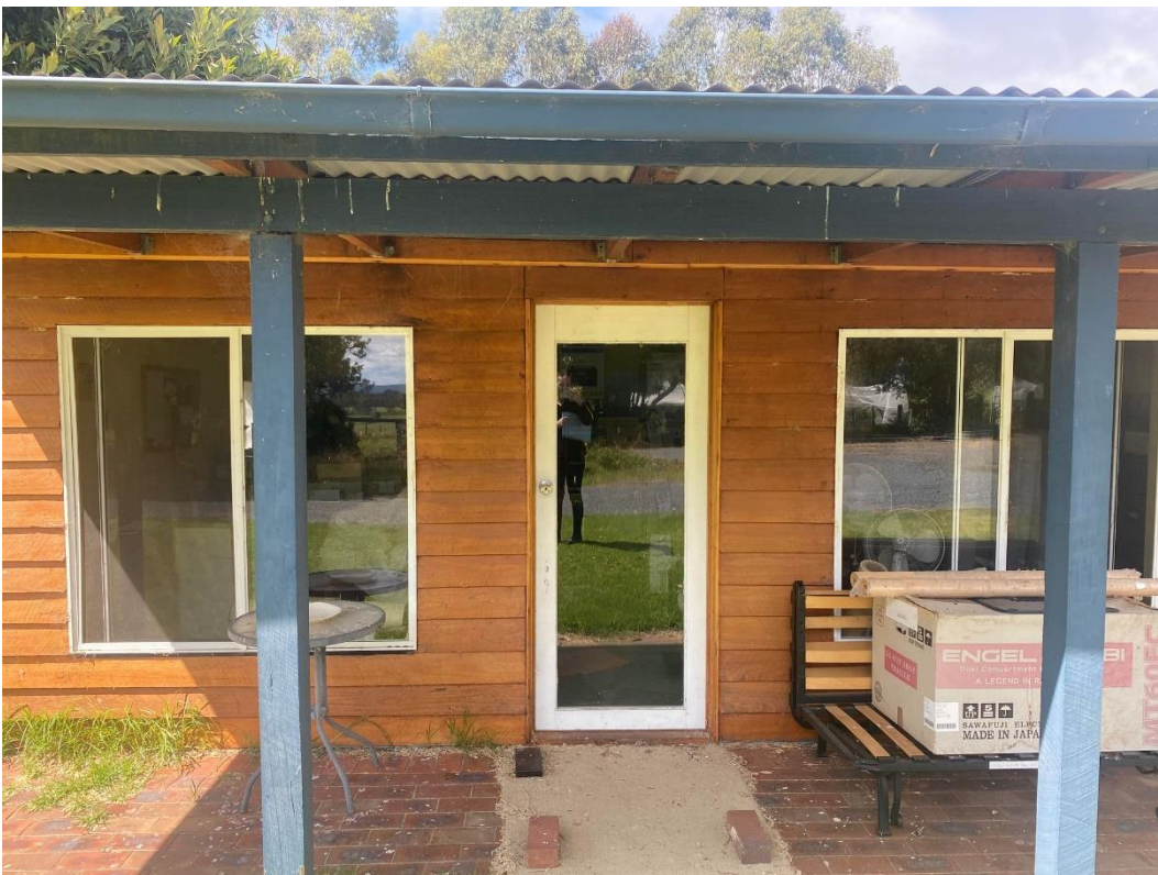
Photograph 2: External photograph of outbuilding
