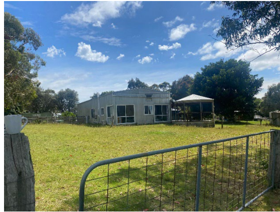
Photograph 10 – Extension to existing dwelling facing north.
