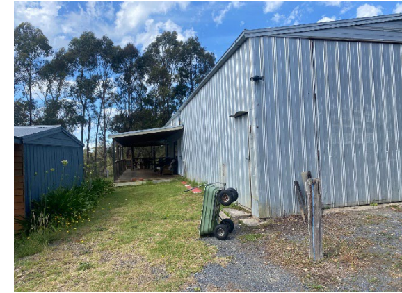
Photograph 6 – Existing extended dwelling showing deck area facing south.
