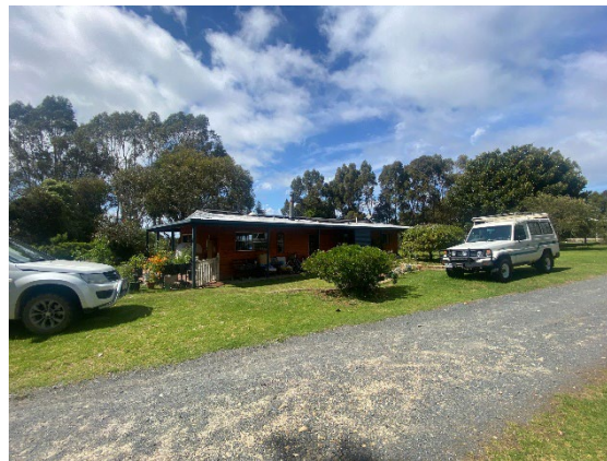
Photograph 5 – Existing dwelling on subject site facing southeast.
