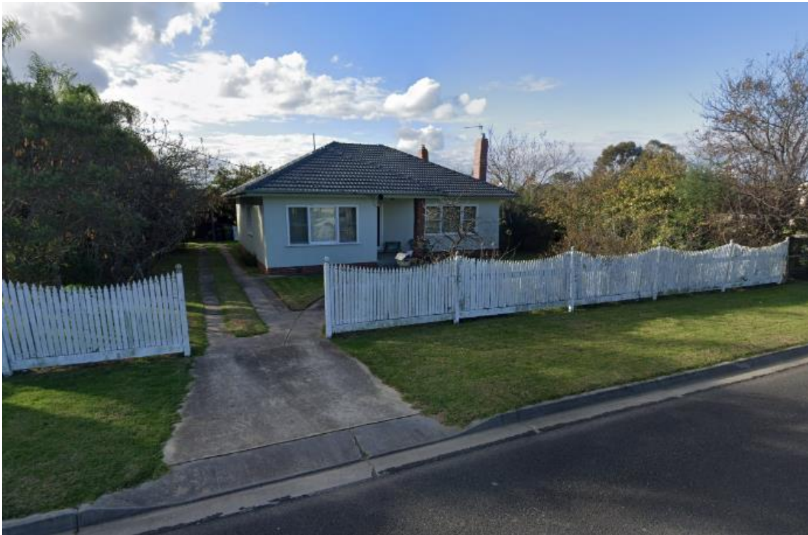
Photo 5: Streetscape image of 131 Princes Highway
