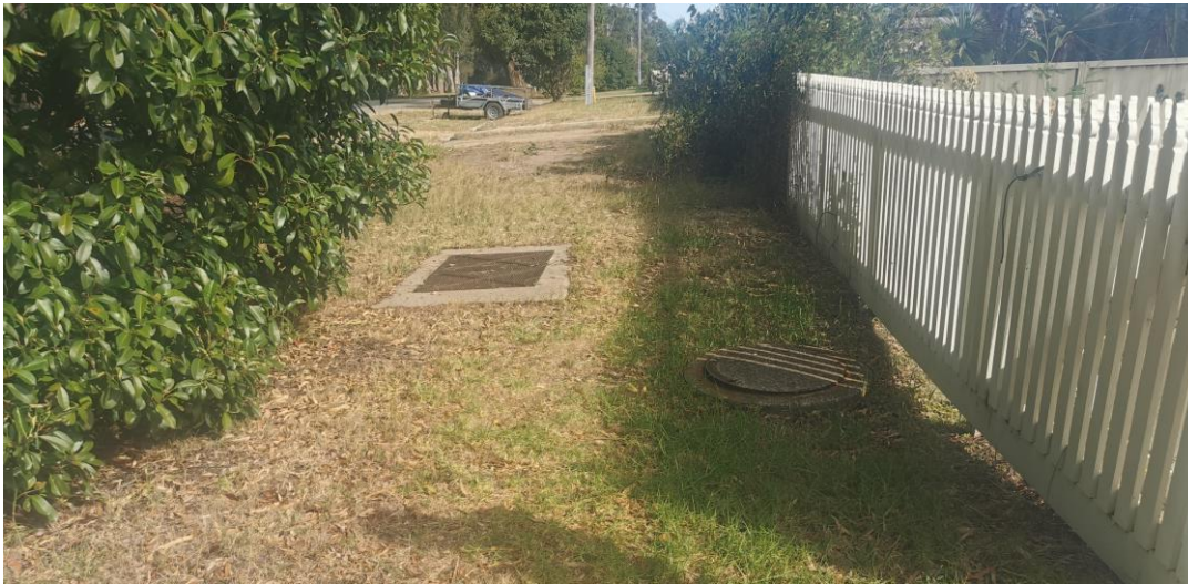
Existing telecom pit and sewer manhole within the adjoining Road Reserve
