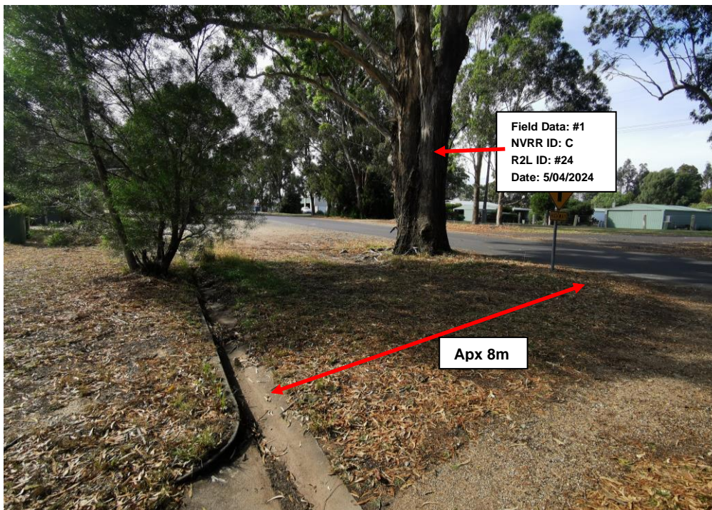
Existing barrier kerb within Punt Road
