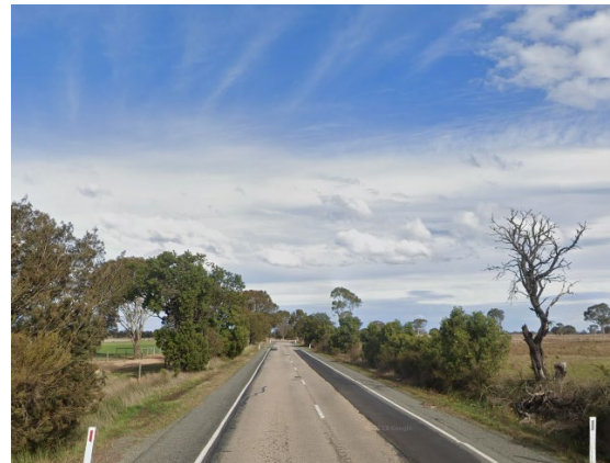
Photograph 17 – Bengworden Road facing south.
