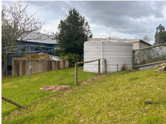
Photograph 8 – Existing water tanks on subject site.
