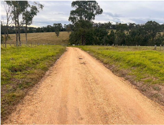
Photograph 20 – Orchard road facing north.
