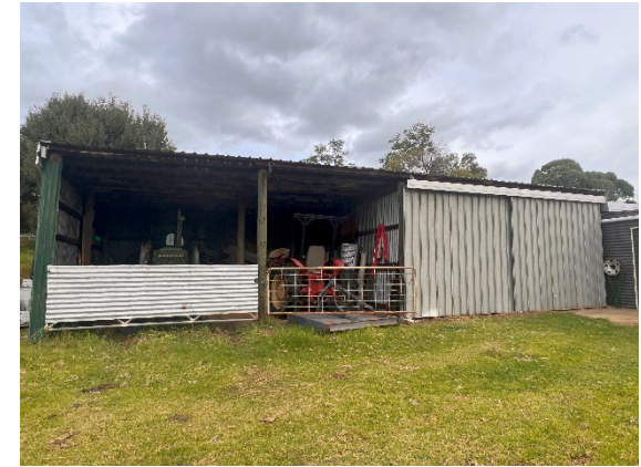
Photograph 6 – Existing outbuilding on subject site.
