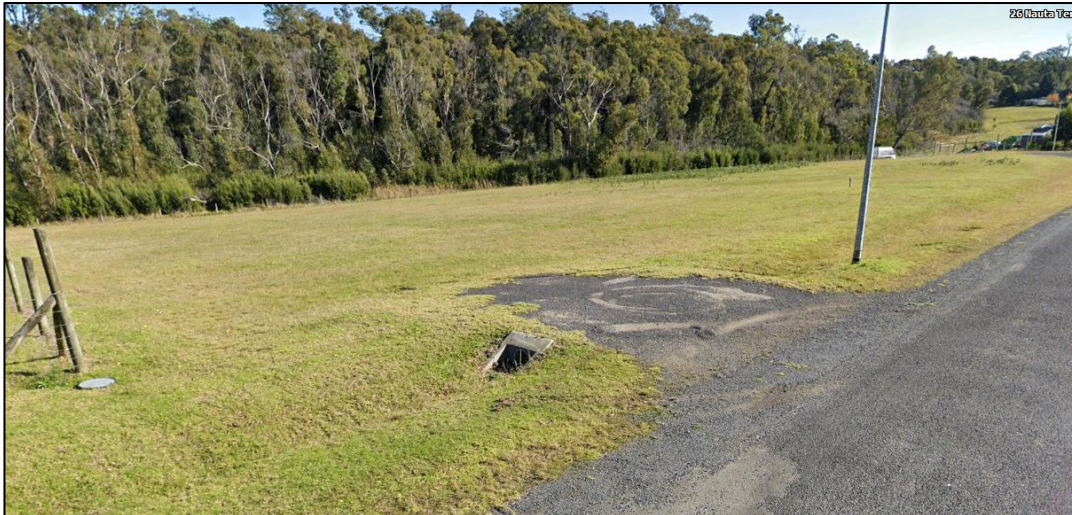
Subject land existing vehicle crossing
