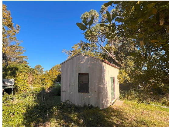
Photograph 10 – Existing outbuilding on subject site facing southwest.
