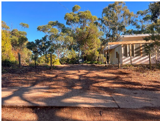
Photograph 3 – Existing driveway entrance to the subject site and proposed Lot 1.
