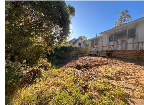
Photograph 6 – Proposed Lot 1 facing north along the western boundary.
