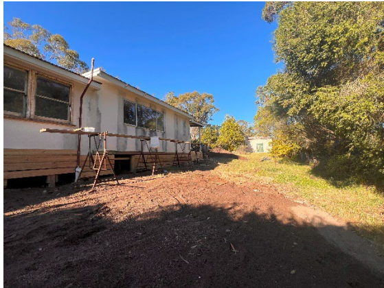
Photograph 8 – Proposed Lot 1 facing south.
