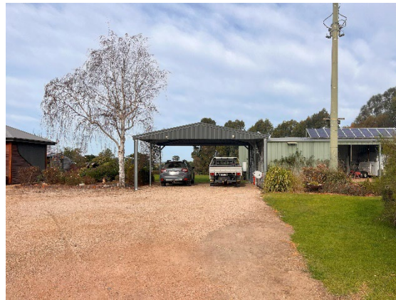
Photograph 5 – Existing carport on subject site facing south.
