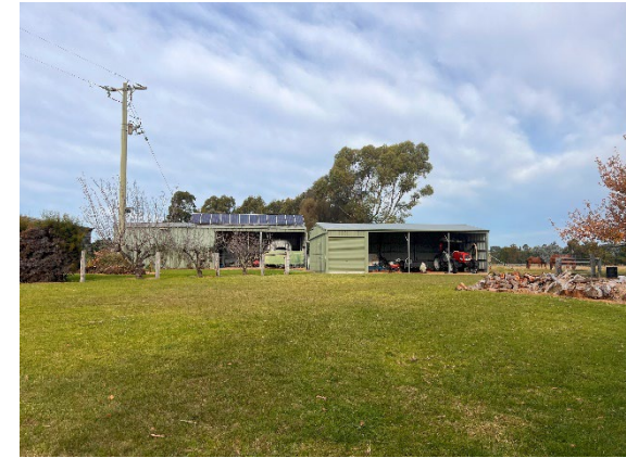
Photograph 6 – Two existing outbuildings on subject site in proximity to the existing dwelling facing south.
