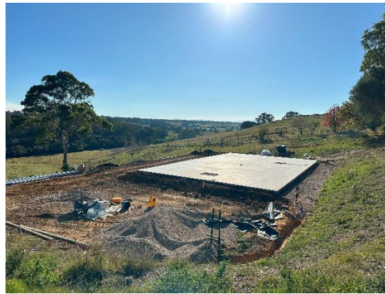
Photograph 5 – Existing dwelling under construction on subject site facing north.
