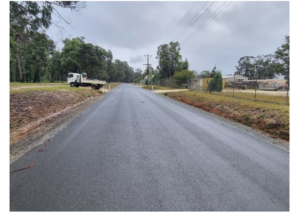
Photograph 12 – Bastion Point Road facing northwest.
