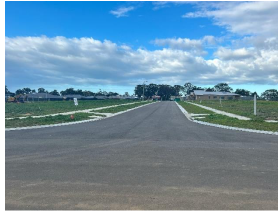
Photograph 16 – Blake Avenue facing south.
