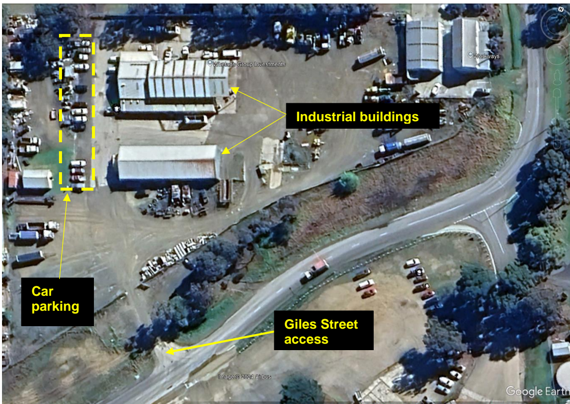
Image of subject land (Google Earth 31/08/2023)
