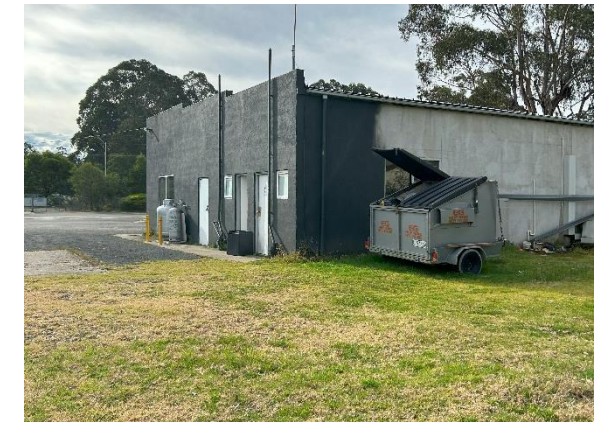
Photograph 7 – Proposed Lot 1 facing north along the western boundary.
