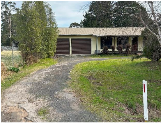
Photograph 8 – Southern access point to proposed Lot 2 facing west.
