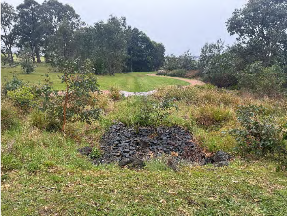
Figure 16: Raingarden / Culvert outfall
