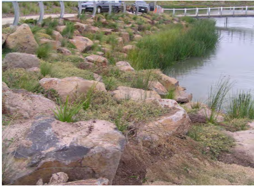
EXAMPLE 2 : STEPPED ROCK BASIN PLANTED BATTER
