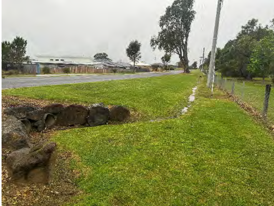
Figure 14: External catchment toward Boyd Court
