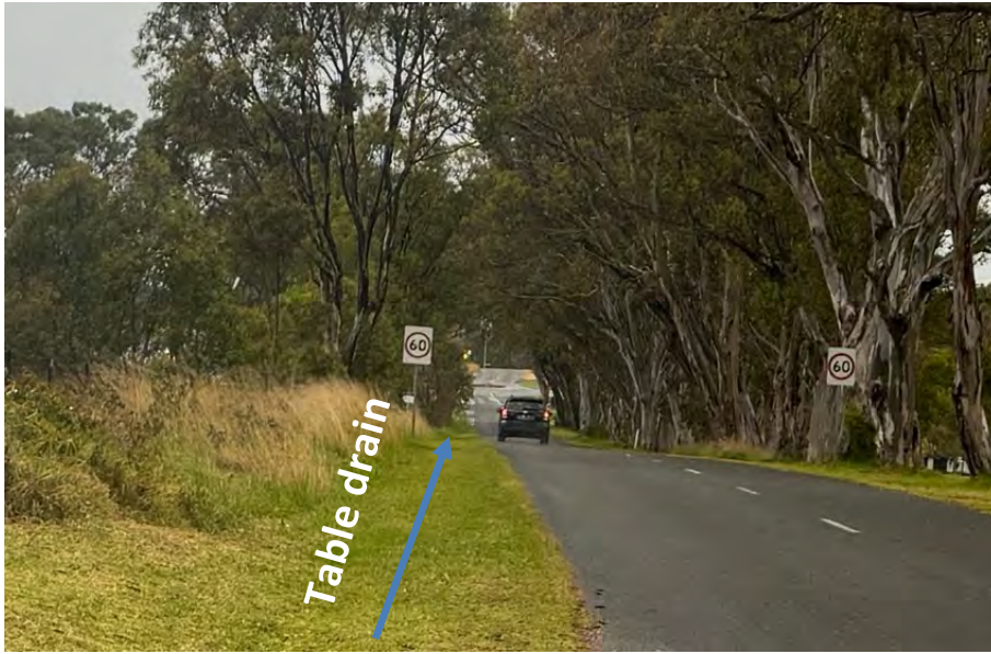
Figure 10: Eagle Point Road Table Drain
