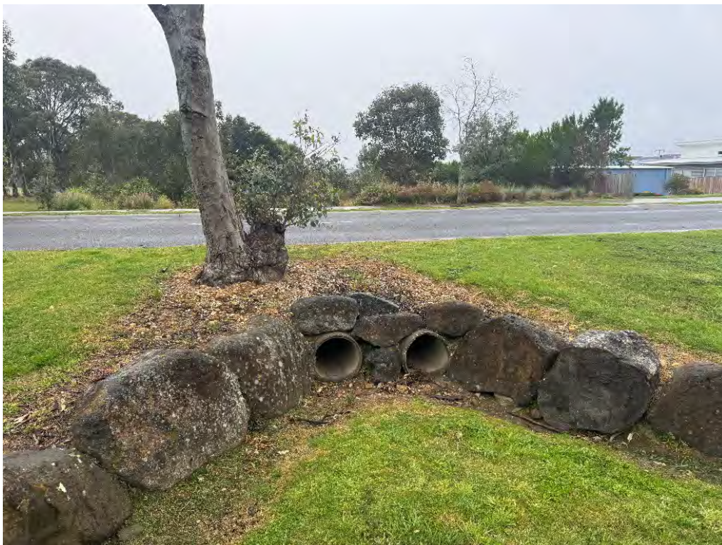
Figure 15: EPR twin culvert
