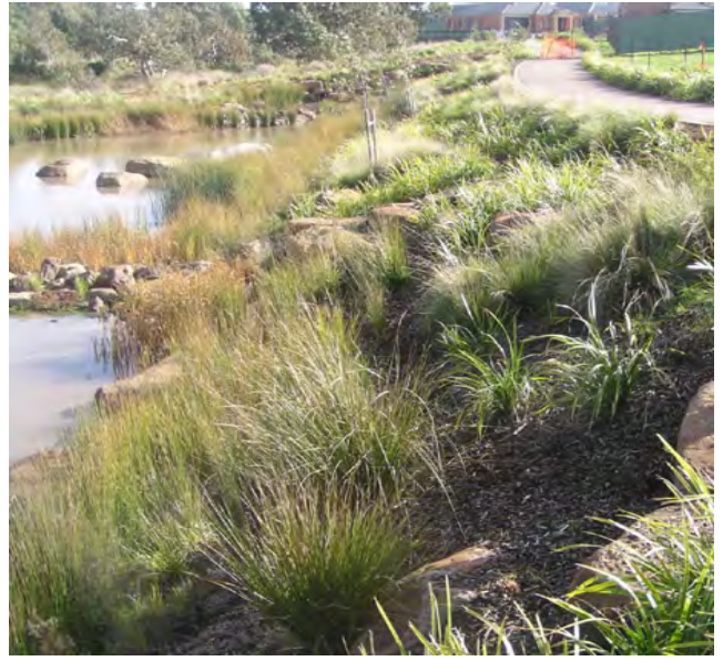
EXAMPLE 1 : STEPPED ROCK BASIN PLANTED BATTER
