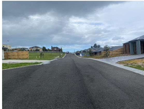
Photograph 17 – Lakeview Drive facing east.
