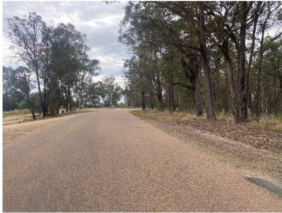
Photograph 14 – Mount Lookout Road traversing southeast.
