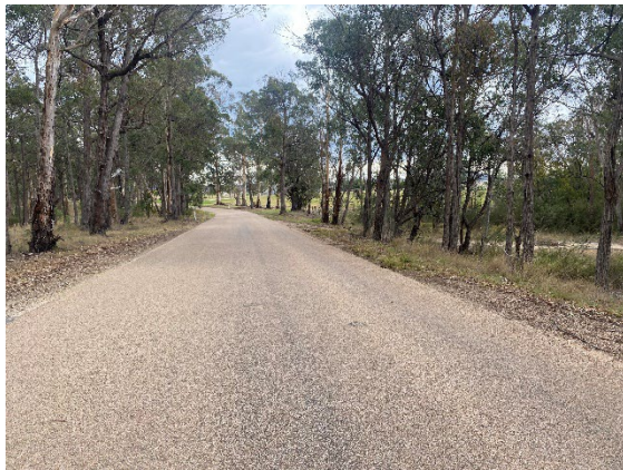
Photograph 15 – Mount Lookout Road traversing northwest.
