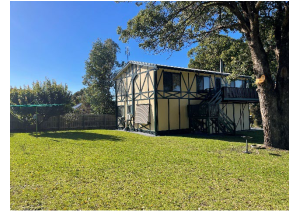
Photograph 6 – Proposed Lot 4 facing southeast.
