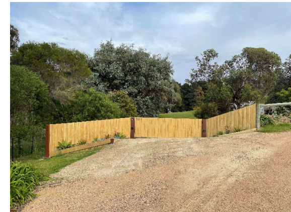
Photograph 7 – Existing access to 18 Lakeshore Drive.
