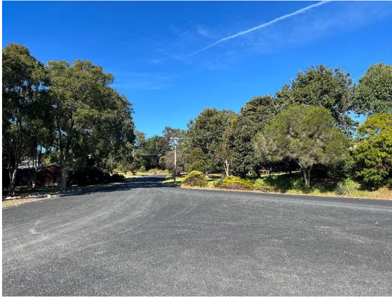
Image of Lawriel Court looking south
