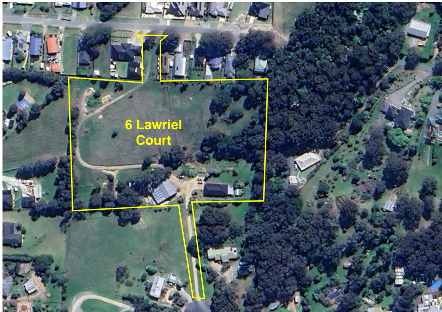
Aerial image of the northern neighbouring property of the subject land being 6 Lawriel Court (Source: Google Earth)
