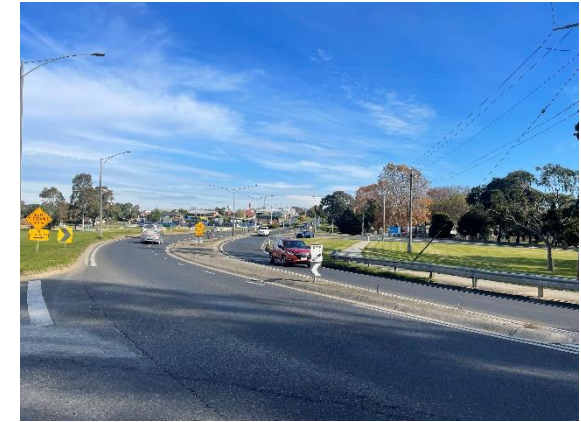
Photograph 16 – Main Street facing west.
