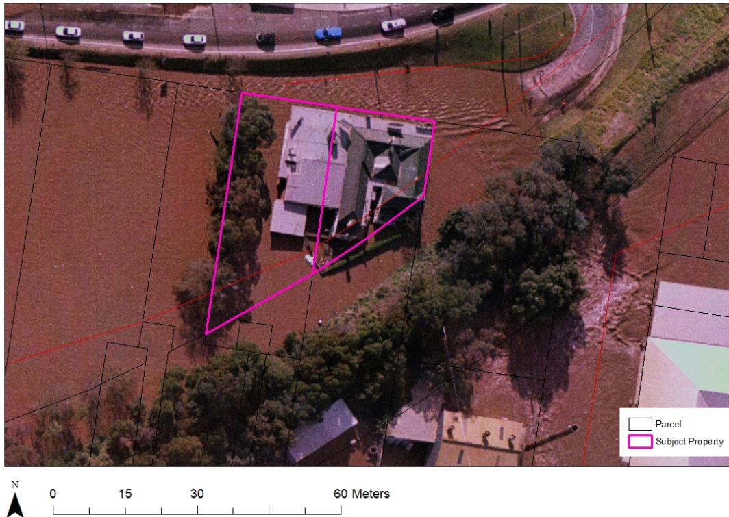
Figure 2 – June 2007 flood event
