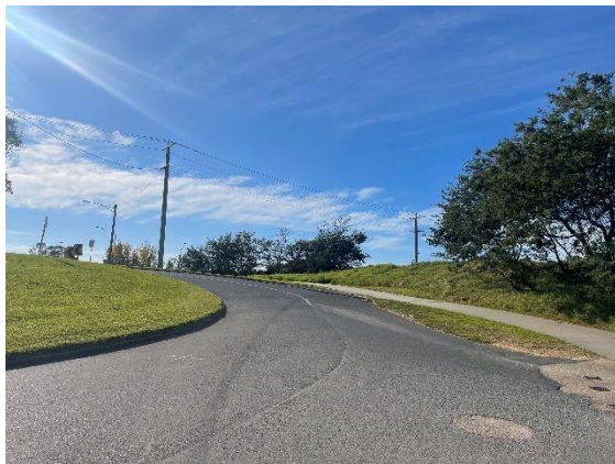
Photograph 7 – Existing access road to subject site facing northeast.
