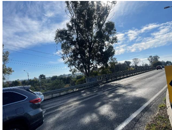
Photograph 15 – Main Street facing east – Mitchell River Bridge.
