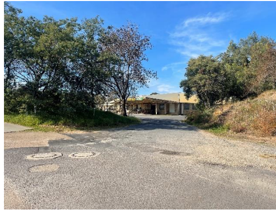
Photograph 14 – Neighbouring property at 2 Macleod Street, Bairnsdale southeast of the subject site.
