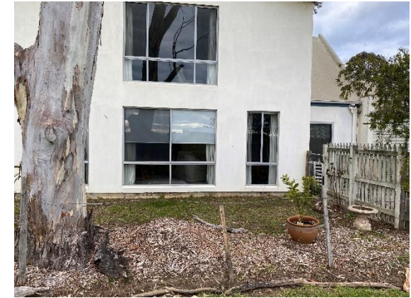
Photograph 6 – Proposed Lot 2 facing south showing current boundary.
