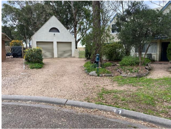
Photograph 2 – Existing driveway entrance to the subject site at 11 Woodland Court, Paynesville.
