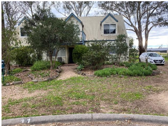
Photograph 3 – Southern side of 11 Woodland Court facing north showing existing dwelling.
