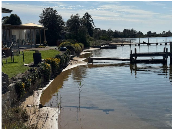
Photograph 3 – Proposed location of boardwalk adjoining residential land facing northeast.
