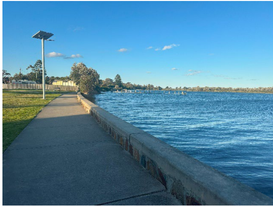
Photograph 2 – Existing concrete footpath facing east showing Cunninghame Arm.
