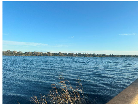
Photograph 11 – Existing concrete footpath facing southwest showing Cunninghame Arm.
