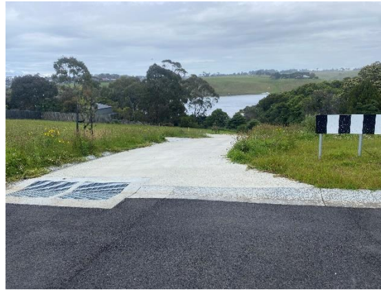
Photograph 16 – Lakeview Drive facing west.
