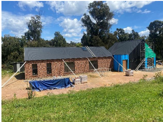
Photograph 3 – Existing dwelling on subject site, to be contained on proposed Lot 1.
