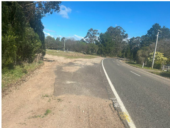
Photograph 21 – Secondary access to the Great Alpine Road and former bus stop at the entrance to 200 Great Alpine Road, Bruthen.
