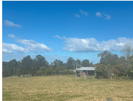
Photograph 11 – Existing 'hay' shed on the proposed Lot 4.
