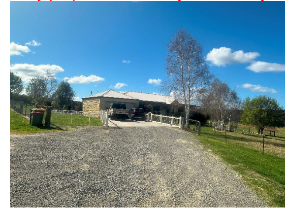
Photograph 6 – Existing dwelling, north on the subject site to be on proposed Lot 1.
