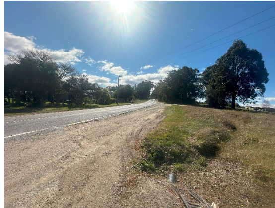
Photograph 22 – Great Alpine Road adjoining the western boundary of the subject site facing north.
