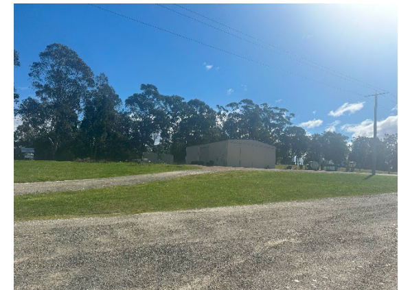
Photograph 7 – Existing outbuilding in northwest corner of subject site to be on proposed Lot 1.
