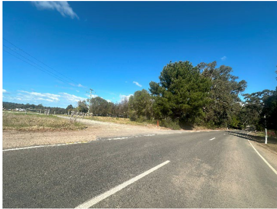
Photograph 2 – Existing driveway entrance to the subject site at 200 Great Alpine Road.
