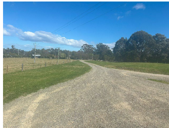
Photograph 5 – North of the subject site, facing southwest showing existing access driveway.
