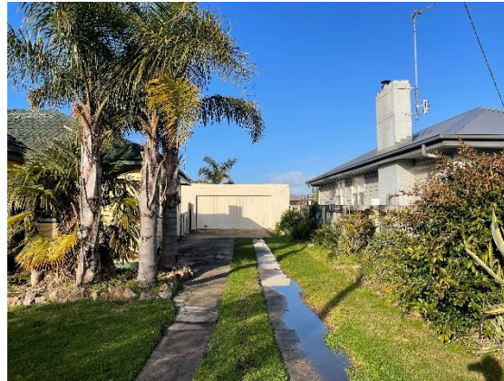
Photograph 4 – Existing driveway access to rear of subject site and proposed Lot 2.
