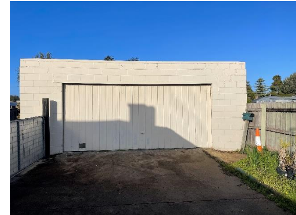
Photograph 6 – Existing outbuilding to be removed on subject site.
