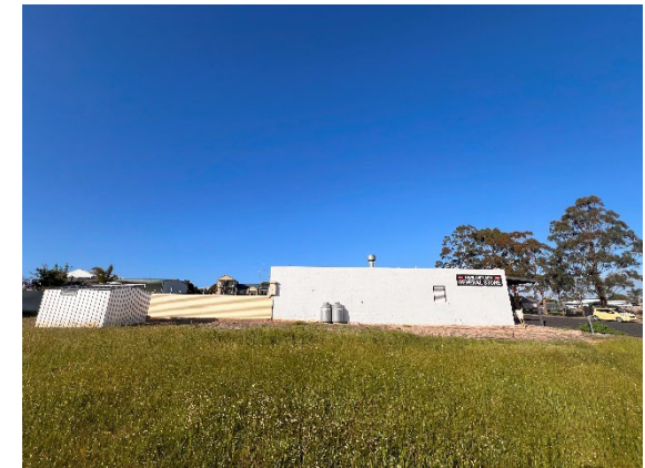
Photograph 7 – Subject site facing southwest.
