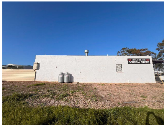
Photograph 11 – Neighbouring property adjoining the southwestern boundary at 10-12 Centre Way, Newlands Arm.
