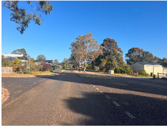
Photograph 14 – Colony Club Drive facing northwest.
