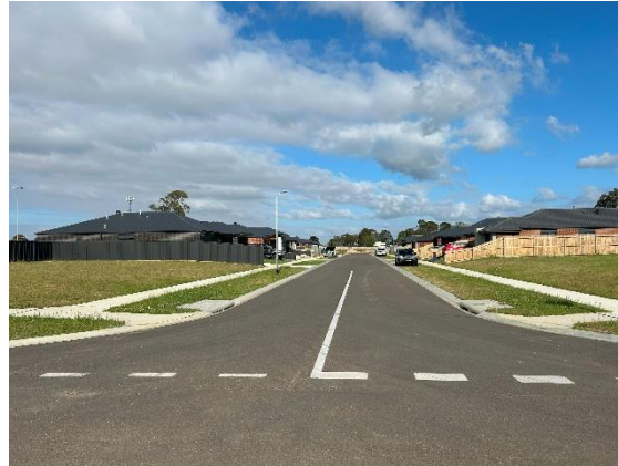
Photograph 17 – Honeyman Avenue facing west.
