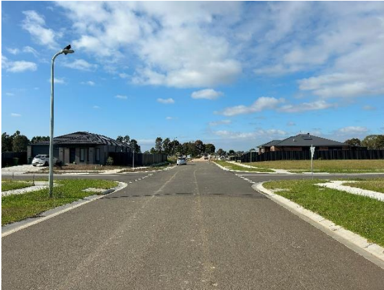
Photograph 15 – Ralston Drive facing south showing intersection between Ralston Drive and Honeyman Avenue.
