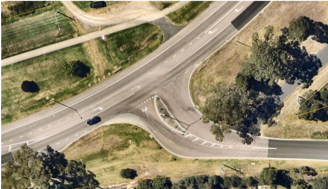
FIGURE 5: AERIAL PHOTO OF PRINCES HIGHWAY / HADFIELD STREET INTERSECTION
