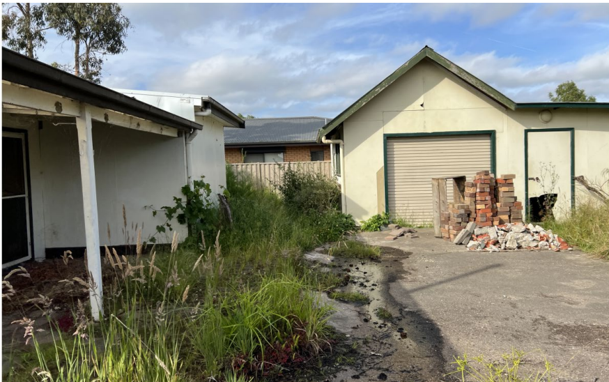
Photograph 4: Looking north across the rear yard of No.22 Alexander Parade
