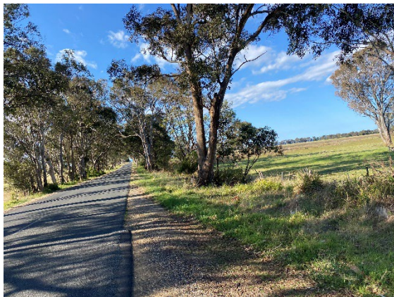
Photograph 15 – Grandview Road facing north.
