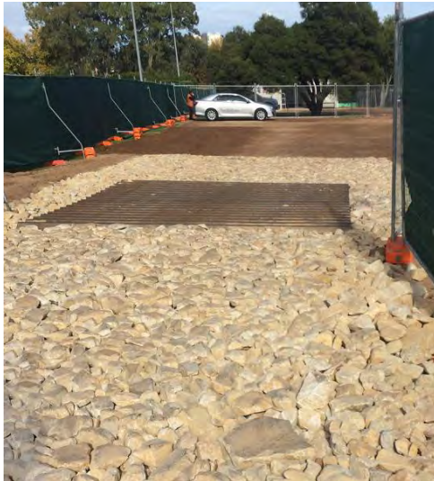
Figure 2. Rumble grid. (photo courtesy of McConnell Dowell)
