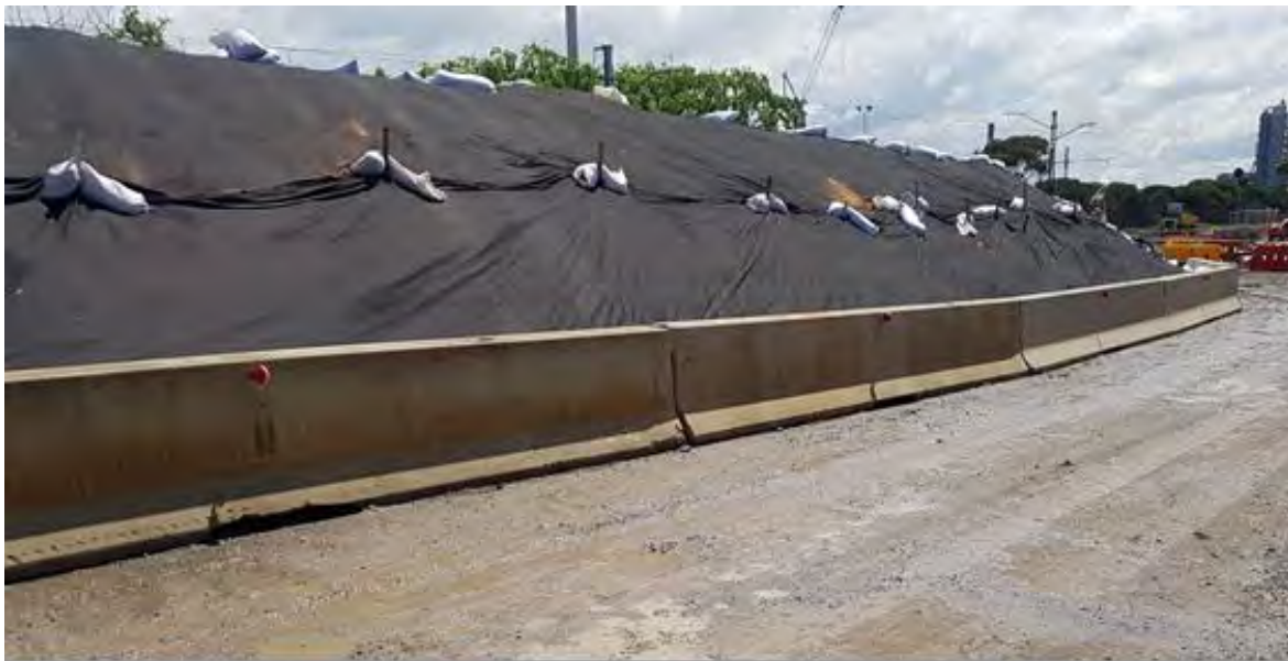
Figure 2. Covered stockpile. (photo courtesy of McConnell Dowell)
