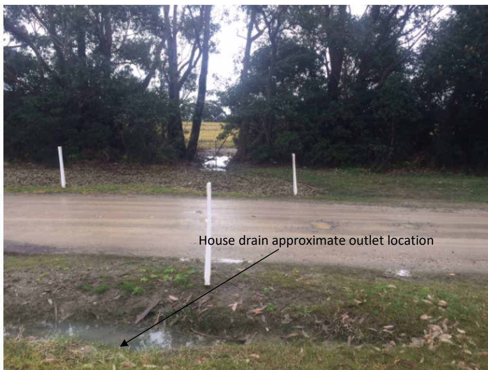
Figure 8: Ward Street house drain outfall
