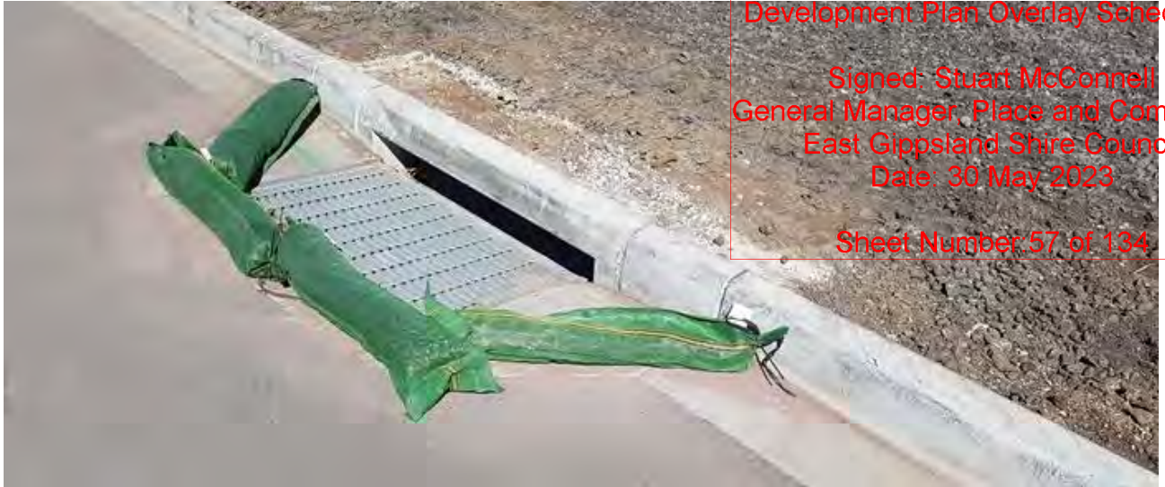
Figure 5.3. Silt sock in use to prevent sediment entering drain inlets. (photo courtesy of McConnell Dowell)
