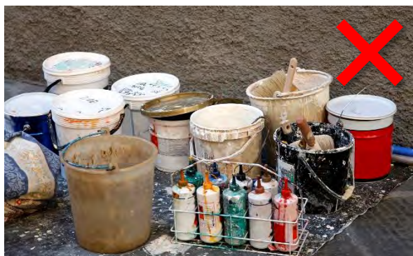
Figure 7.1. Incorrect chemical storage onsite.
