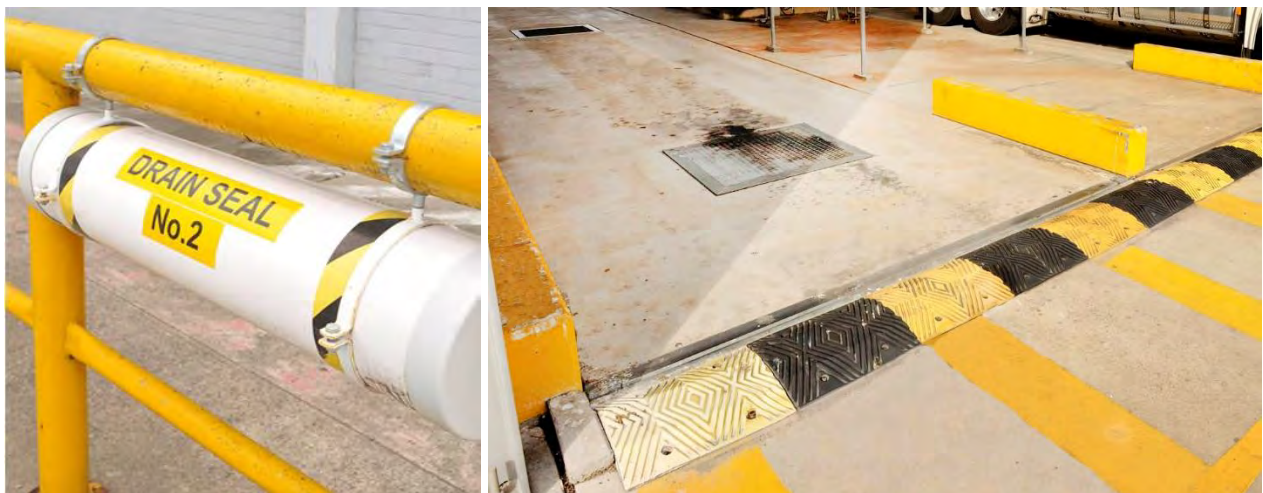
Figure 7.5. Drain seal (left) and rollover bund (right).
