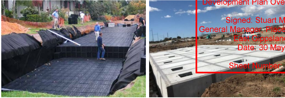
Figure 14: Subsurface Detention Tank examples (under construction) 4
