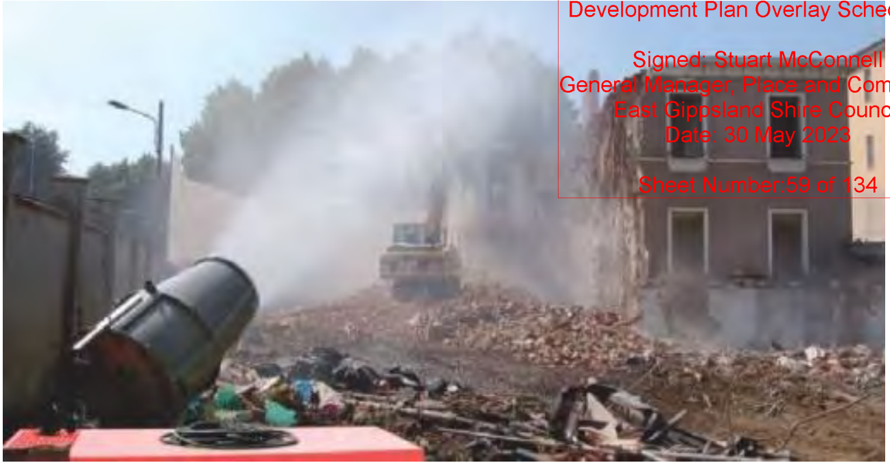
Figure 5.5. Dust suppression using water spray during demolition works. (photo courtesy of Kane Constructions)
