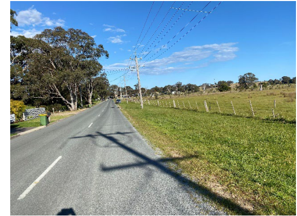
Photograph 12 – Bay Road facing west.
