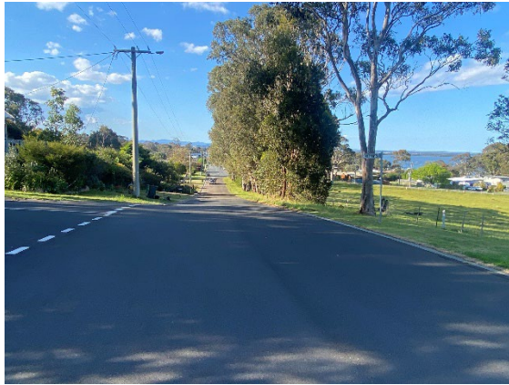
Photograph 14 – Tait Street facing south.
