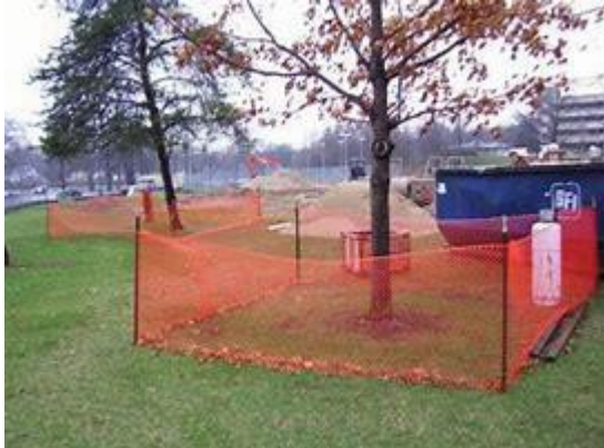
Figure 2 - Either bunting or wire mesh fencing can be used. Flagged rope does not offer enough protection
