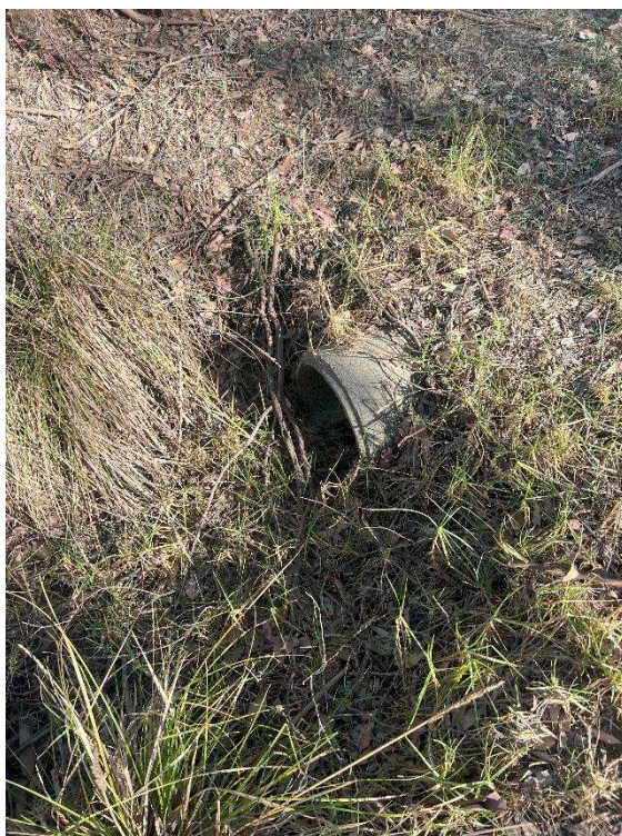
Calvert under Jones Road leading to a swale drain
