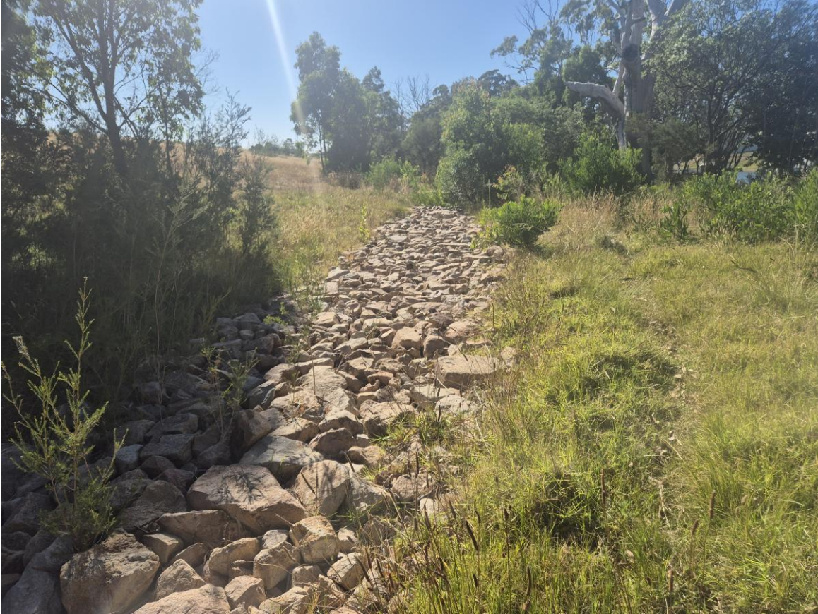
Existing exfiltration drain
