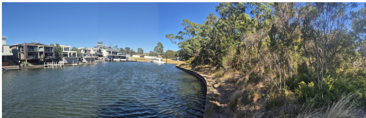
Looking west along revetment wall
