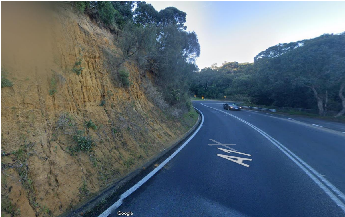
Figure 3-3 Rock Outcrop Observed along Princes Highway (Google Maps)
