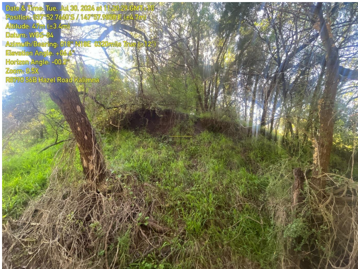
Figure 3-4 Minor Landslide within South West Corner of the Site
