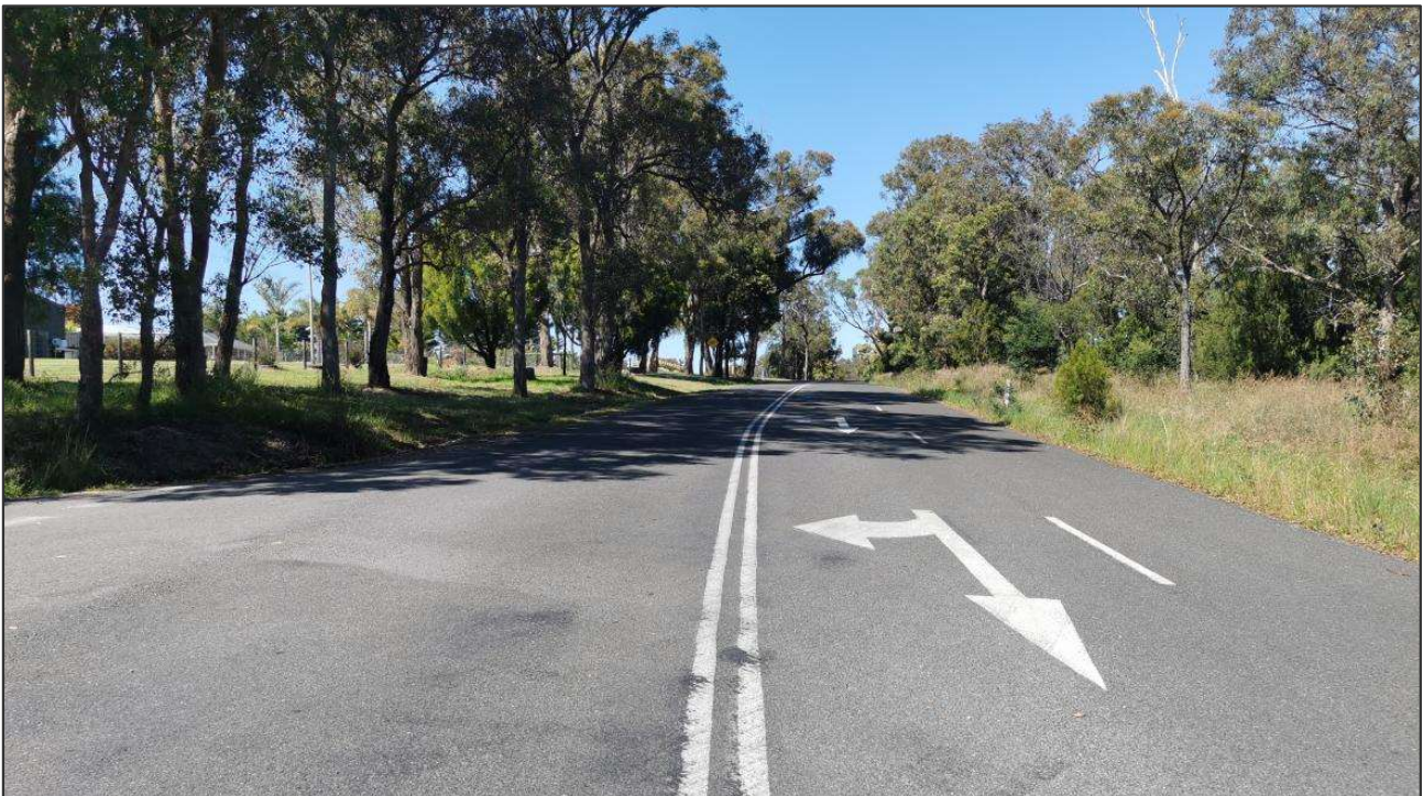
Figure 23 Clifton West Road, AUR treatment at Maclure Drive intersection
